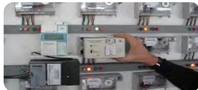
Streetlights and Geyser Ripple Control
